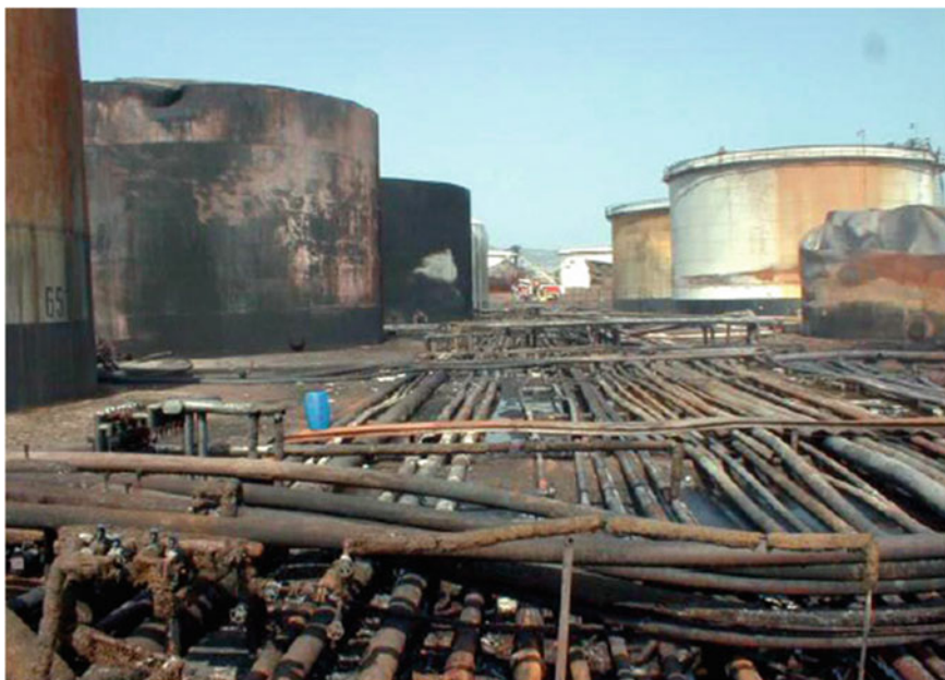
Fig. 13.4 Tüpraş petroleum refinery, fire following the 1999 Marmara (Turkey) earthquake (Scawthorn 2000). Photo by G. Johnson
