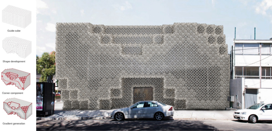
Fig. 24. Hybrid building structure generation
