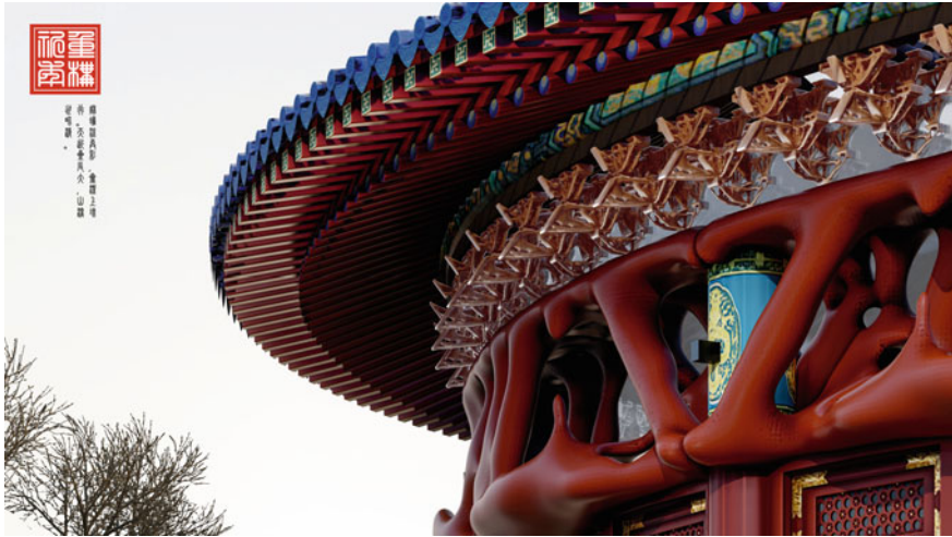
Fig. 11. 3D topological optimized architrave bracket set components
