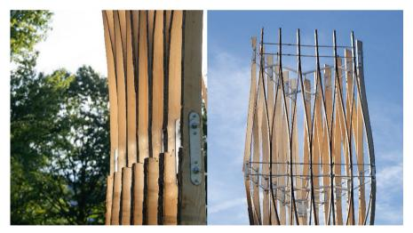
**Fig. 15.** Details of the *UnLog Tower*: finger joint splice connection (left) and robotically kerfed logs stretched along a thread rod (right), photos by Cynthia Kuo..
