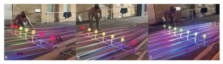
Fig. 14. Object calibration is employed for quality control of prefab wall components.
