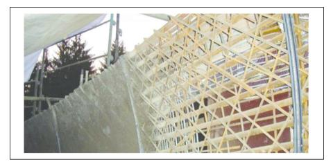
Fig. 2. Oberhof construction of the bobsleigh using shotcrete methods
