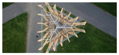
Fig. 9. Reciprocally framed tube steel in the UnLog Tower, photo by Cynthia Kuo.
