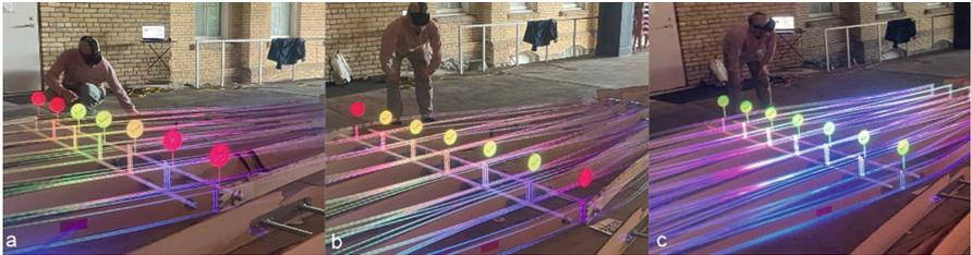
**Fig. 14.** *Object calibration* is employed for quality control of prefab wall components.
