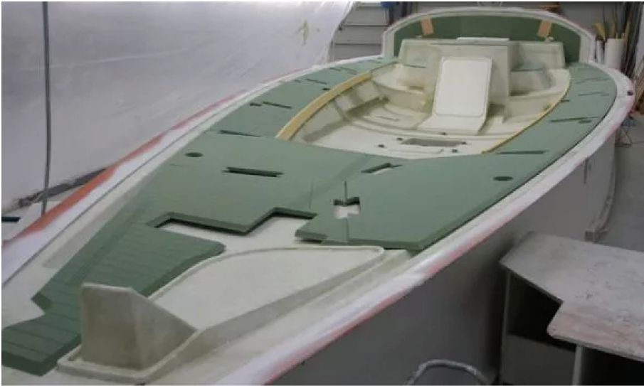
Fig. 1. Typical sandwich construction used in FRP marine vessel manufacturing showing dry fitting a foam core before the final FRP layer is applied (N.B.: the molded deck assembly is commonly inverted during the manufacturing process, as shown). Image from Ricardou (2019).
