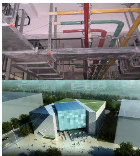
Fig. 16 Setup of the 110-kV ultrahigh voltage Mengzi underground transformer substation of Shanghai World Expo’s fair.
