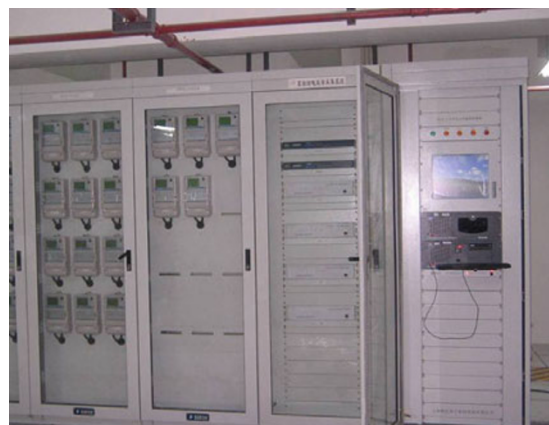
Fig. 17 Mainframe of a distributed fiber Raman photon temperature sensor system.
