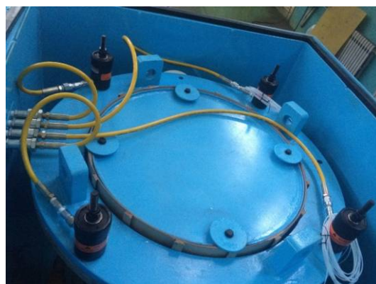
Fig. 7 Field pressure test system of transformer winding.
